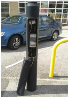
Lighting Column access cover Removed exposing cables
