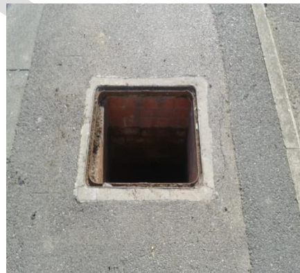
Missing Chamber Cover
